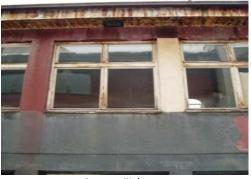
Source Fichtner Figure G-10. Damages on the flashing on roof eaves.
