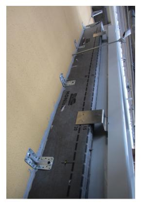
Figure B-25. Windows fastened to the existing facade.
