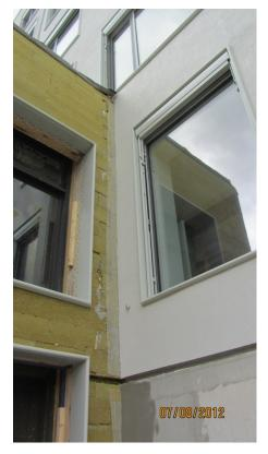
Figure B-26. Insulation and new windows installed.
