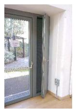
Figure I-14. Manual air intake panel for secure night-purge ventilation.
