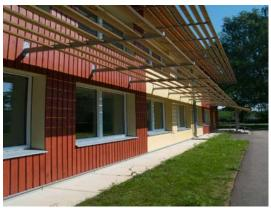
Figure C-6. After refurbishment – overhangs for summer heat protection.
