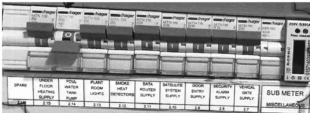
Figure 2 Miscellaneous circuit from main distribution board at Lark Rise
