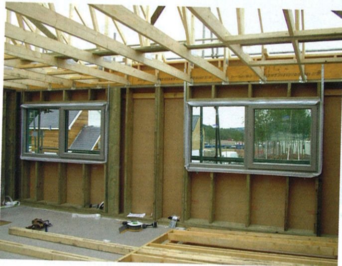
Windows are put in place as the house is constructed.
