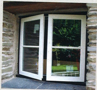
Window at Tyddyn Castell.
